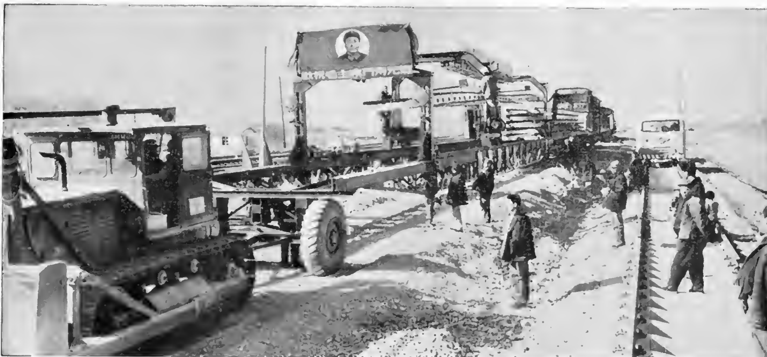
A new rail and tie laying machine designed and made by First Railway Engineering Bureau workers.
